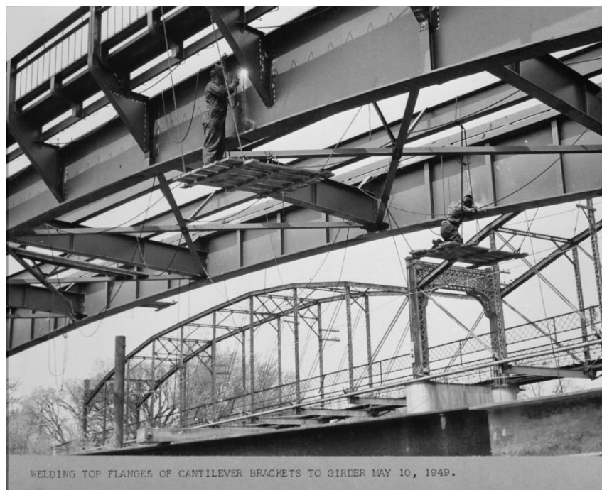
Figure 12. View showing welders at work on both the north and south girders, with the old bridge in the background, looking northwest , around 10 May 1949 (Kallee, n. d.).
