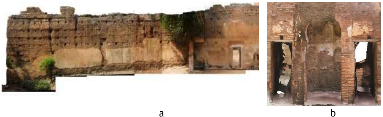
Figure 7. Orthoimages of (a) the North wall (b) the Mihrab (Author's figure).
